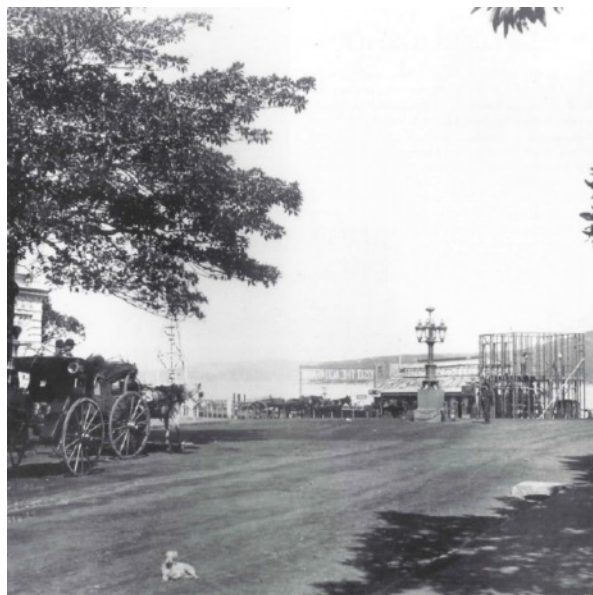
Camera Obscura under construction at Manly Wharf 1888 (NLA)
